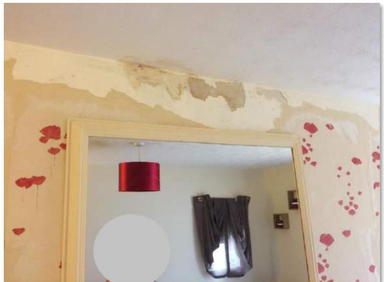
Damp can penetrate through walls and roofs to cause damage inside the building. Overflowing guttering, leaking outflow pipes, missing roof tiles and cracked render can all be culprits.
