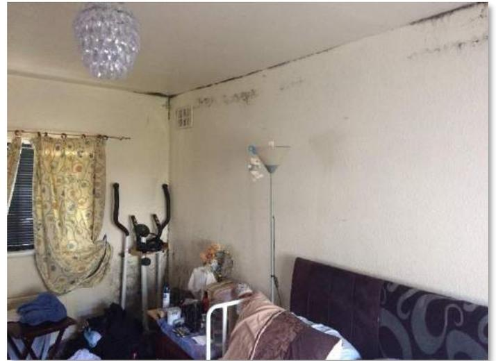
Airborne moisture which comes from breathing, cooking, showering etc can lead to condensation and mould forming in cold corners and on cold surfaces.
