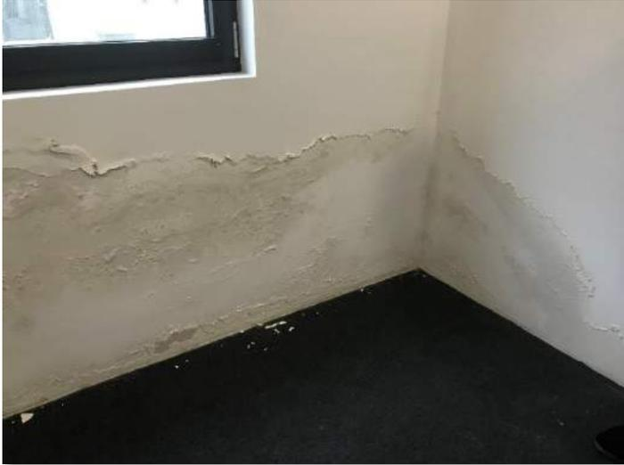
Salt contamination causes blistering on the plaster surface.
